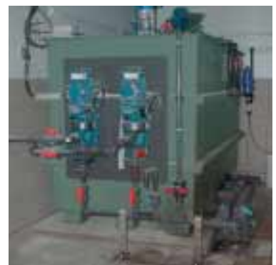
Reagent pumping - polymer injection - lime milk pumping - transfer of activated charcoal
